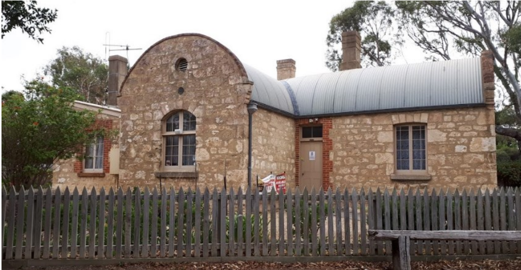
Figure 20. The Railway Superintendents cottage
