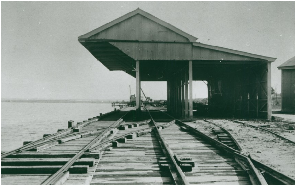
Figure 18. View of the wharf shed with the complicated rail system on the wharf deck to allow for cross overs, 1910 (SL SA B 17516|
