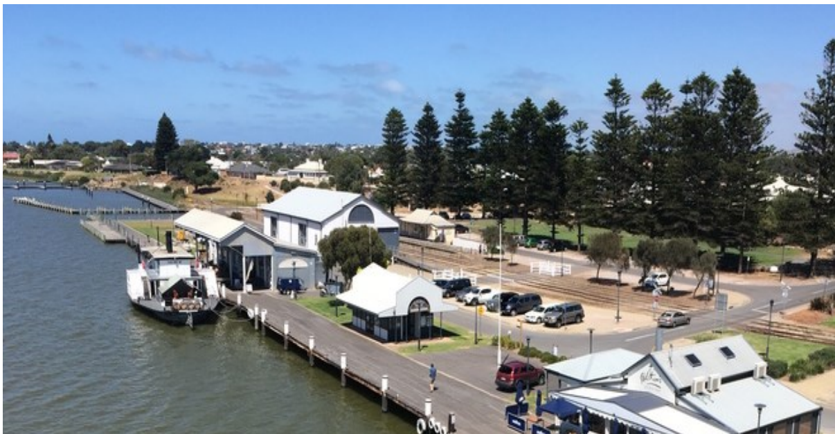
Figure 19. View of the adapted wharf precinct with the remaining rail tracks on the western side running along the railway station.
