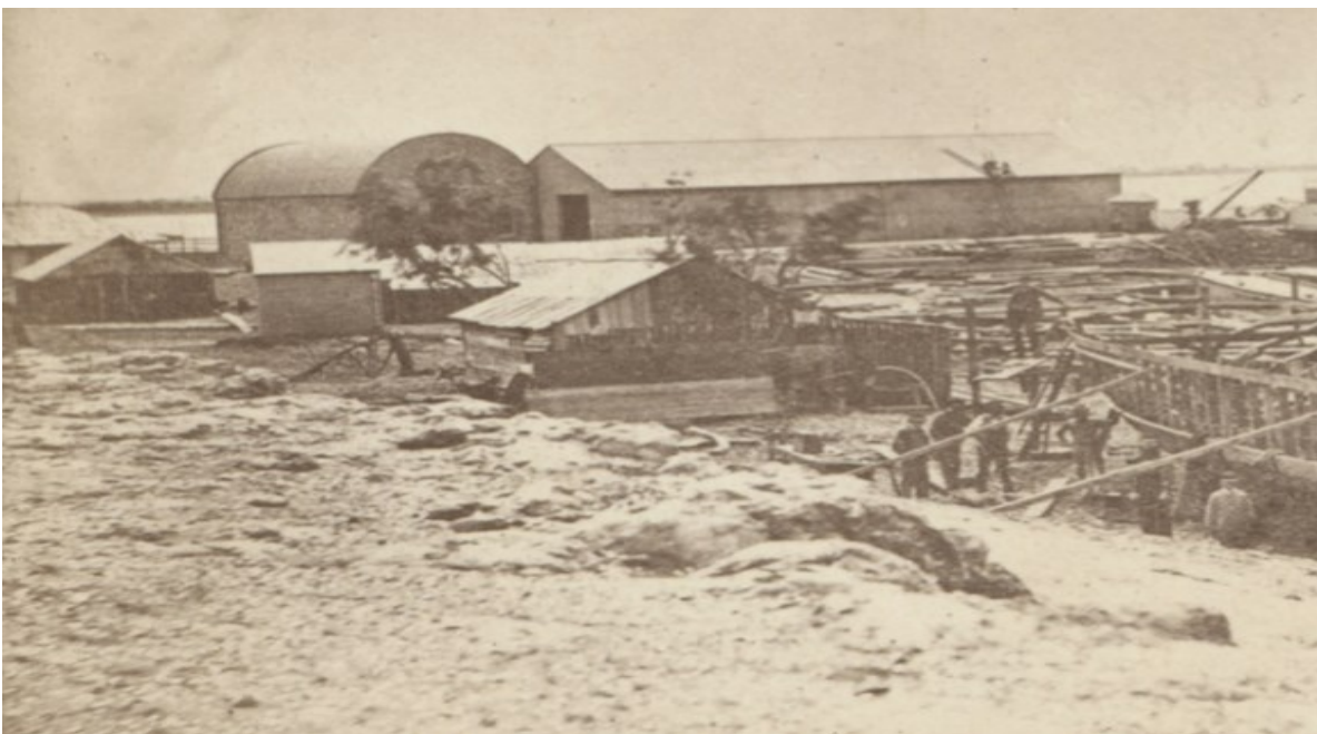
Figure 26. Detail from an image dated to 1866 showing the Government Bond Store with its distinctive curved roof |SLSA B25772|
