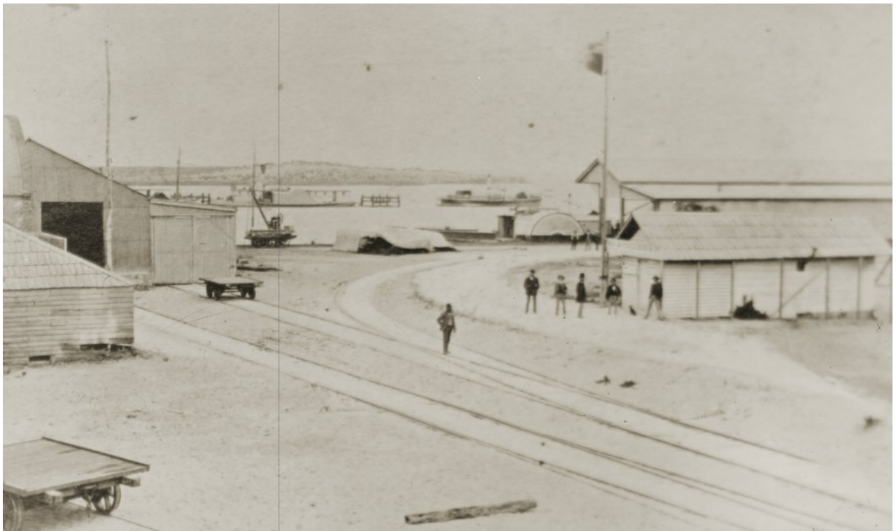
Figure 17. Goolwa wharf with the rail lines coming in from the town; the wharf shed in the background c. 1900 |SLSA B100004|
