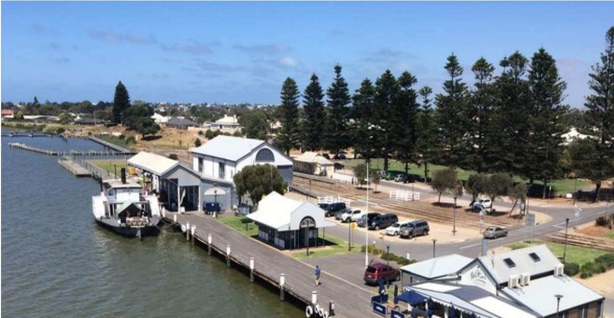
Figure 31. View of the adapted wharf shed and new deck
