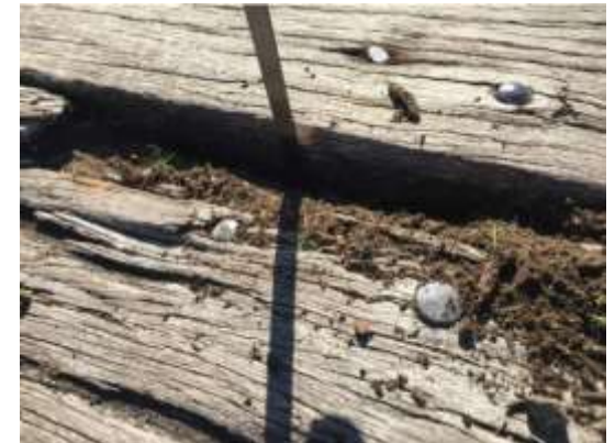
Image: Example of timber degradation of the Goolwa Wharf
