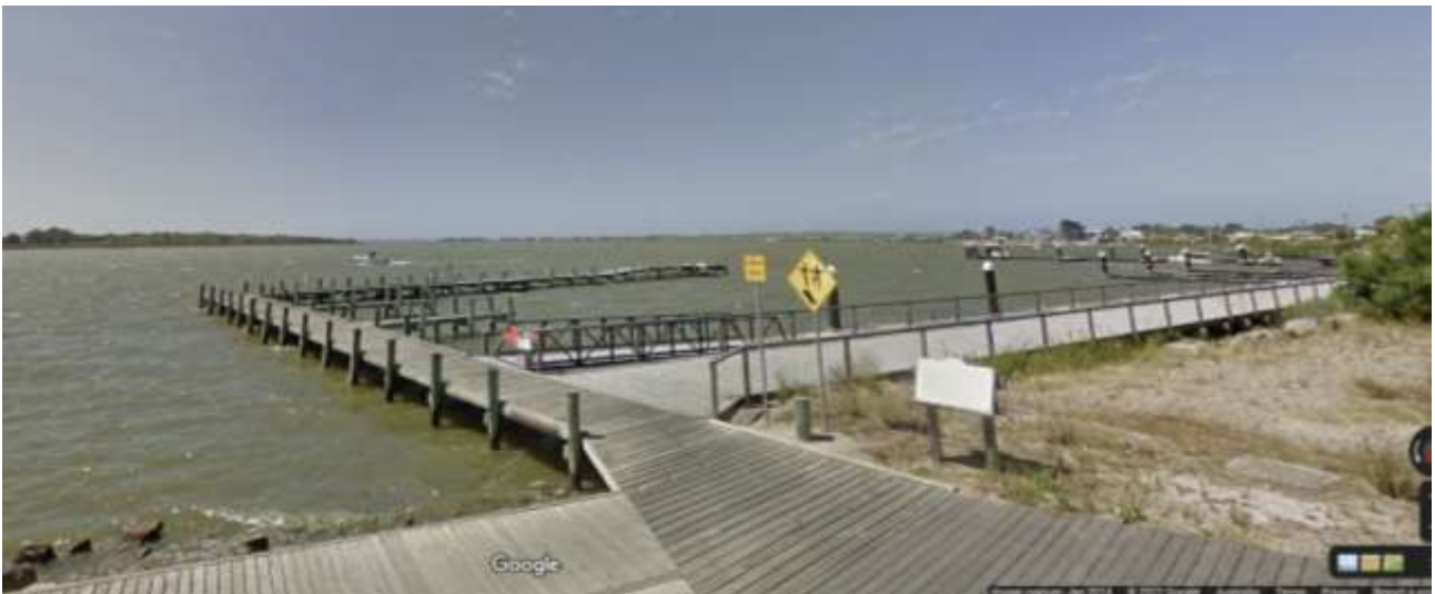
Figure 14: Existing Mooring Facilities (located immediately south of the Wharf Precinct)
