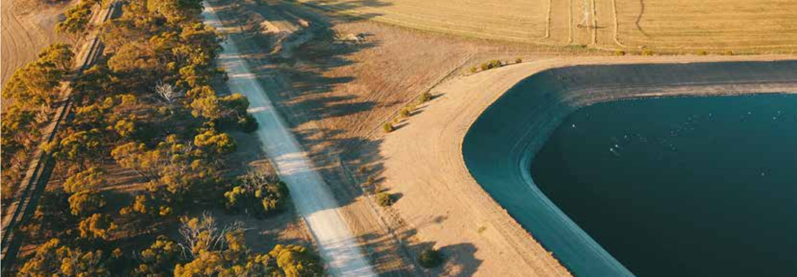
Wastewater treatment plant, Strathalbyn
