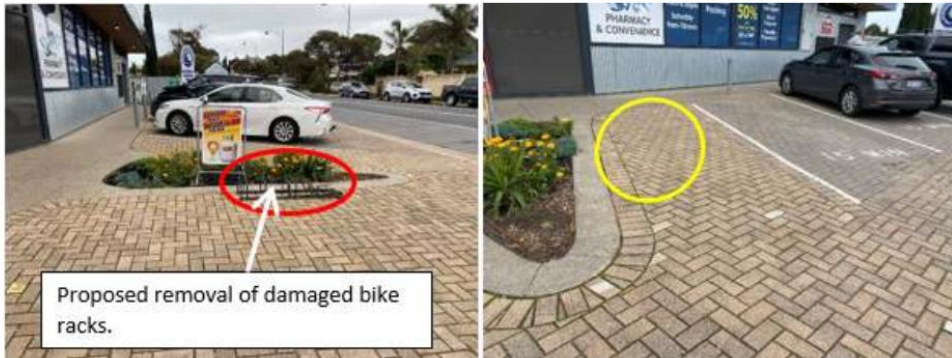
Removal of old bike racks that were hit by a vehicle, and suggested location for new bike racks outside IGA.
