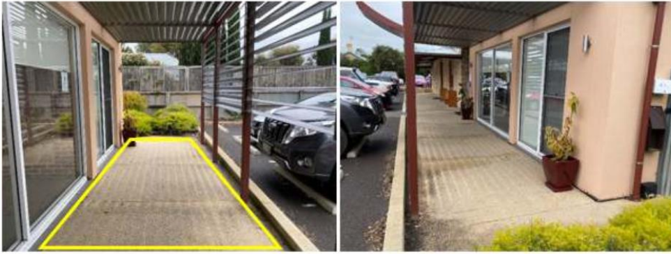
Preferred location for bike racks at Mill House Medical Centre.
