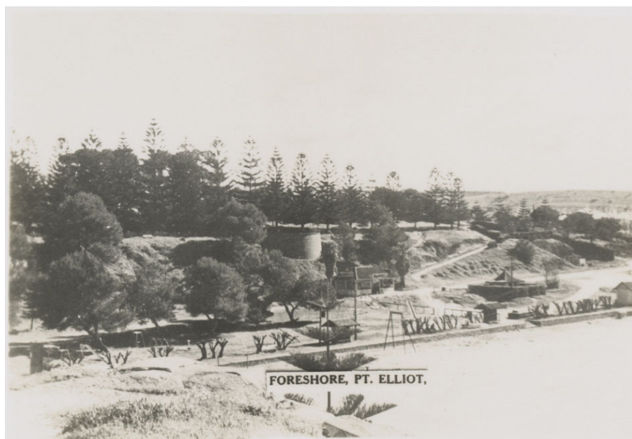
Figure 18: The next major intervention was the construction of a sea wall from the western end of the bay to the bowling club. The probable purpose was to provide separation of the reserve and the beach, and not to provide protection from actions of the sea. Source: State Library of SA.
