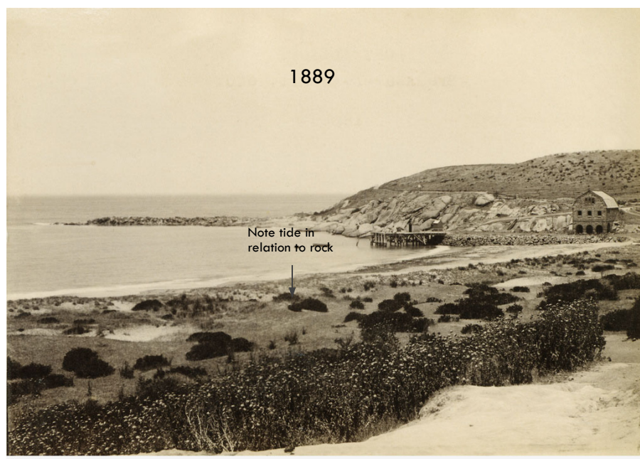
Figure 15: First intervention was installation of breakwater, jetty, and stone walling. The breakwater changed the way in which wave action interacted with the bay. Photograph taken in 1889 from what is now the Blue Dolphin Holiday Apartments.
