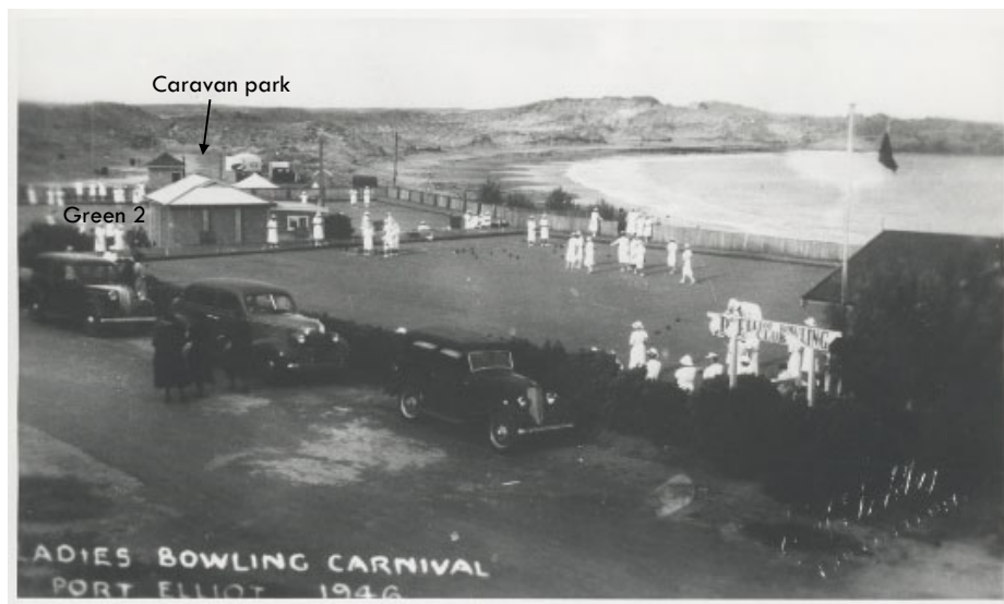
Figure 20: By 1946, the bowling greens had been constructed in their current locations. The caravan park began in this era also on the eastern side of the bowling green. (State Library of SA)
