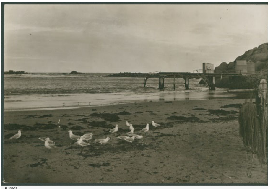
Figure 43. The point of this comparison is to quantify changes to the breakwater. Note the lower section at the end of the breakwater. The archives say that blocks were dislodged in the first storms, and perhaps this was the location. Note that the breakwater in 1942 is almost 'level top' aligned with the former jetty. Source: State Library, permissions pending.
