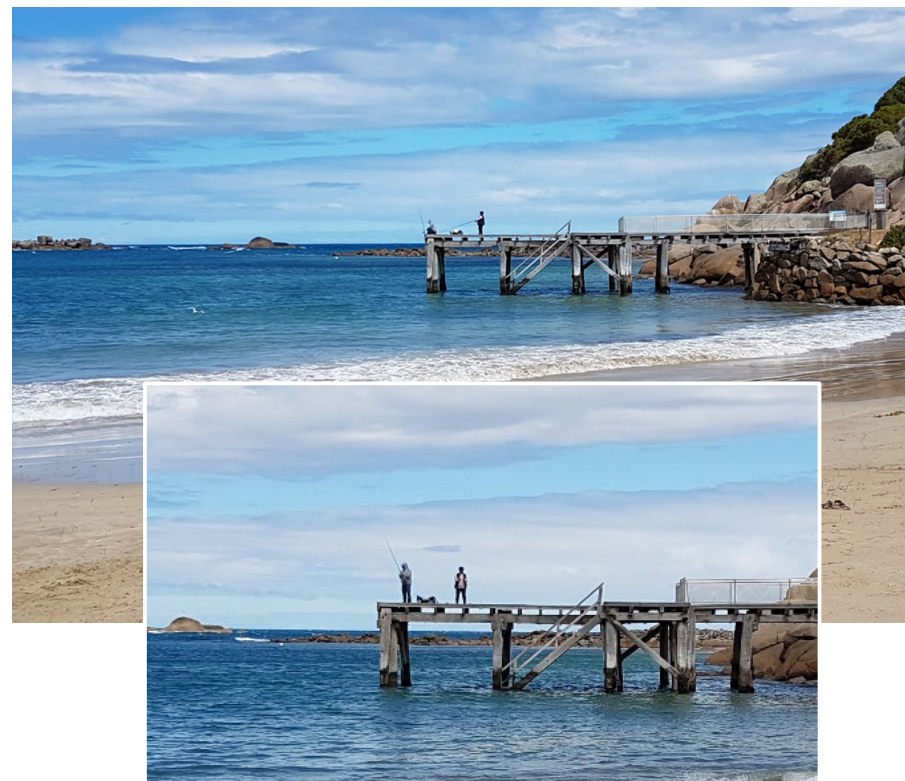
Figure 43. The point of this comparison is to quantify changes to the breakwater. Note the lower section at the end of the breakwater. The archives say that blocks were dislodged in the first storms, and perhaps this was the location. Note that the breakwater in 1942 is almost 'level top' aligned with the former jetty. Source: State Library, permissions pending.
