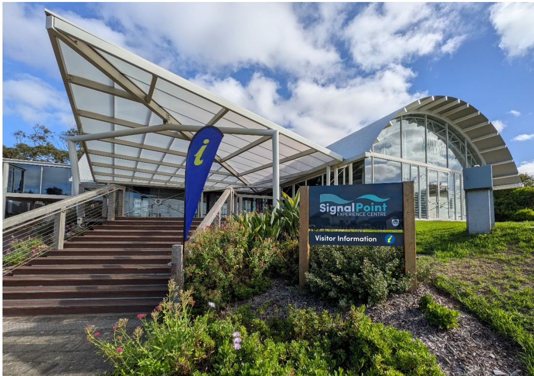
Photo 3: The state-of-the-art Signal Pont Experience Centre.
