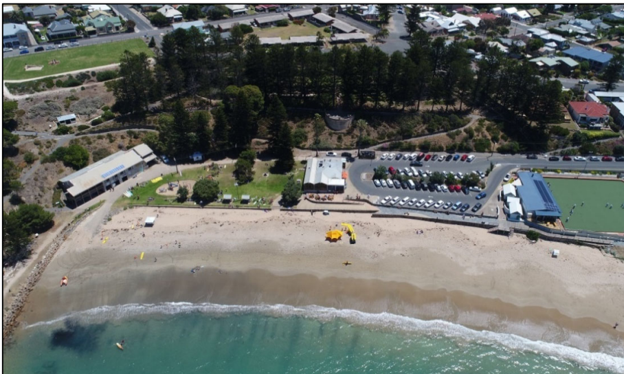
Figure 11: Seawalls at Horseshoe Bay have altered the nature of the backshore
