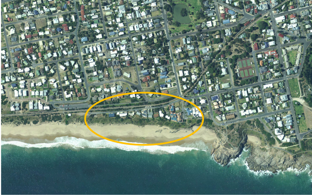
Figure 58: Private development situated on the foreshore (cliff) at Boomer Beach (east)
