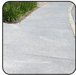
Exposed Aggregate Concrete Footpath
