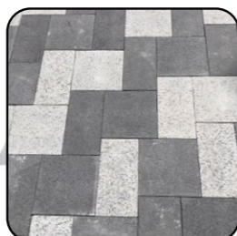
New Footpath Paving
