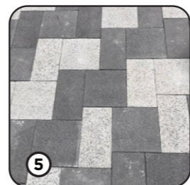
New Footpath Paving
