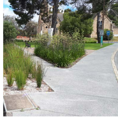
Exposed aggregate footpaths Exposed aggregate footpaths matching from Sunter Street works will be continued through to Swale Street intersection
