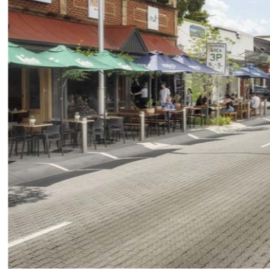
Traffic calming Raised paved intersections will slow vehicles travelling down the street providing a safer environment for pedestrians
