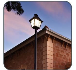
New Street Lighting
