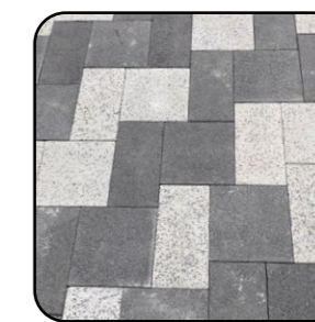
New Footpath Paving
