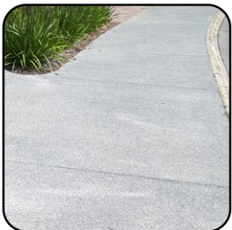
Exposed Aggregate Concrete Footpath
