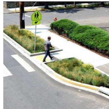
Planted protuberances Additional planting will be used through new protuberances. These could also be used for water sensitive urban design
