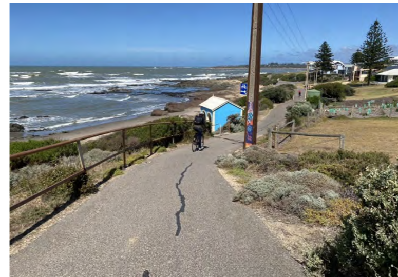
Existing steep section at Middleton Point
