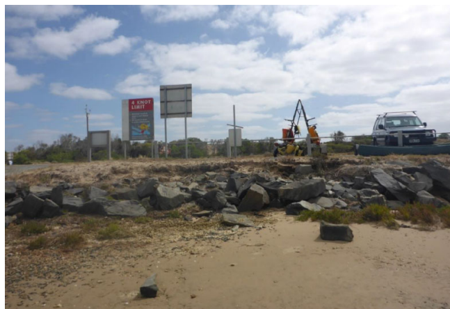
Figure 10- Existing seawall adjacent the eastern side of the boat ramp.
