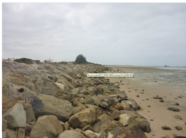
Figure 13- Older seawall east of the boat ramp carpark.
