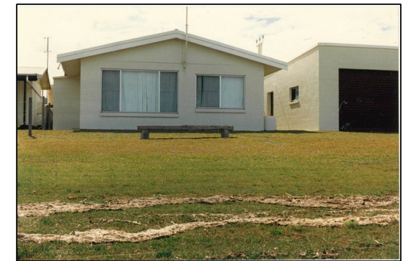
Figure 11: Tidal lines on low-set blocks (19790000)
