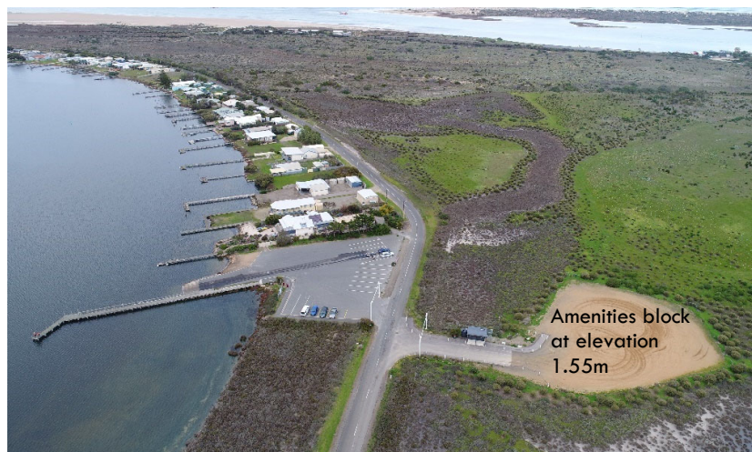
Figure 24: Boat ramp facility and public amenities block.
