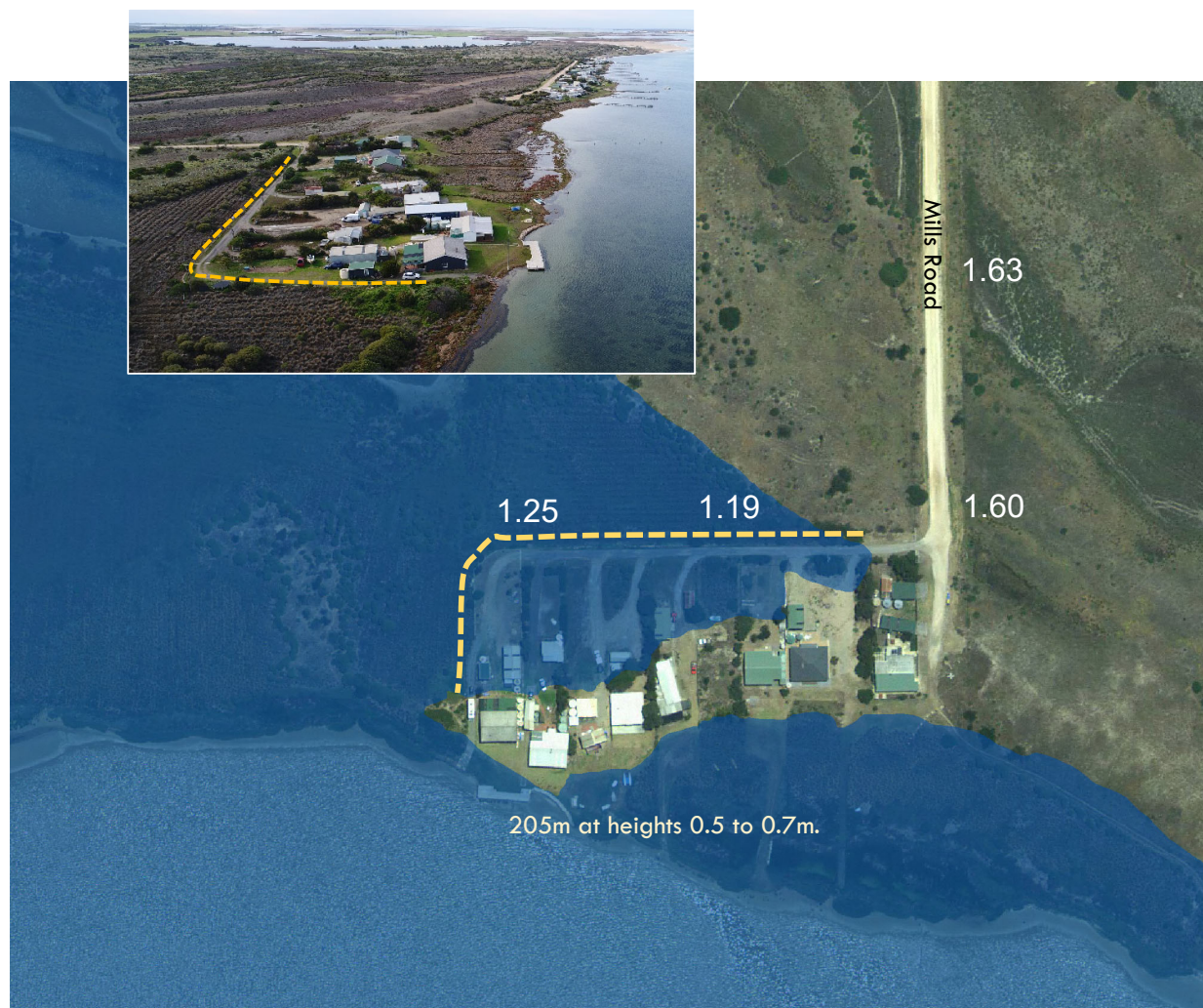
Figure 49 Modelling indicates that internal access to Mills Road settlement would be vulnerable to flooding in the current 1 in 100-year ARI event.
