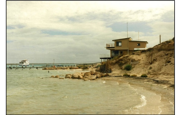
Figure 10: Erosion occurring on Sugars Beach in 1979 (19790000)
