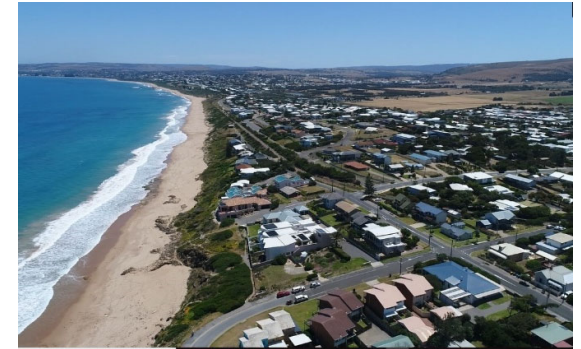
Figure 2: The Goolwa to Victor Harbor railway line dissects the backshore of Boomer Beach
