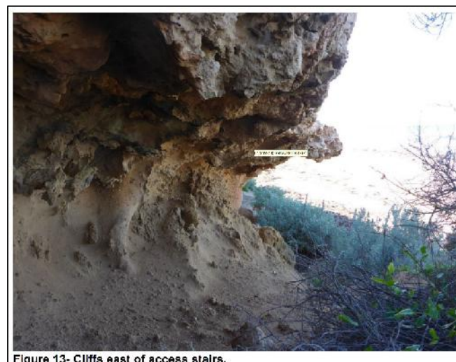
Figure 13- Cliffs east of access stairs.
