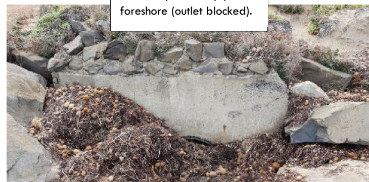
Left: Note the scouring from storm water outflow (DEM 2018). Impacts from storm effects will be greater in locations where the beach has been lowered. Sea level rise will exacerbate the problem.
