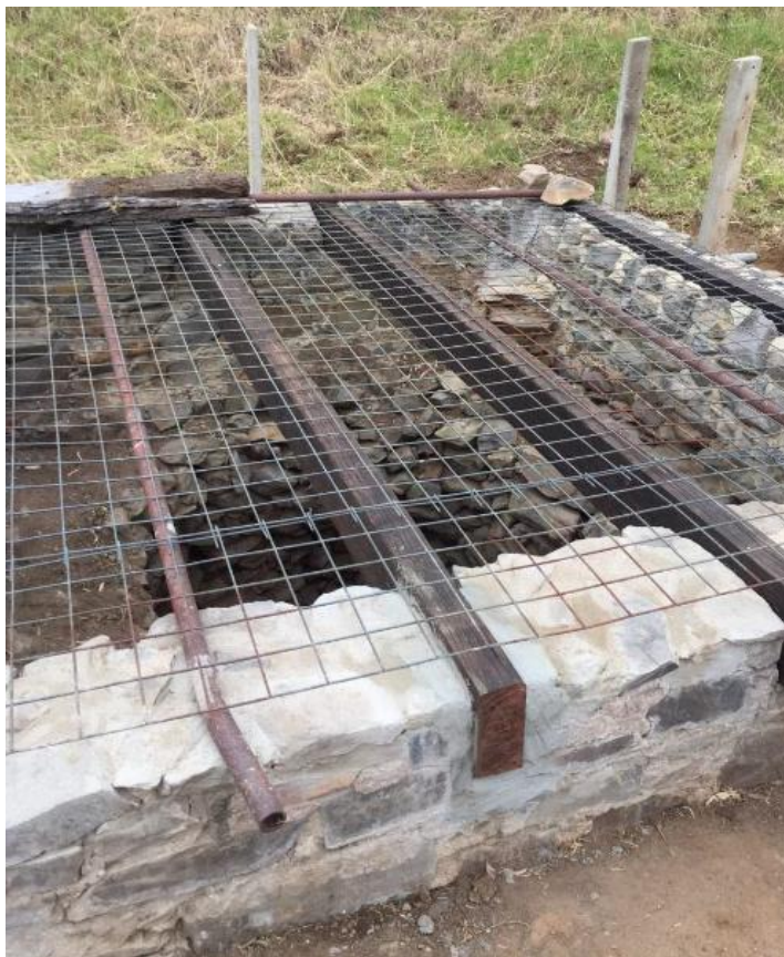
Restoration of Mary's Well
