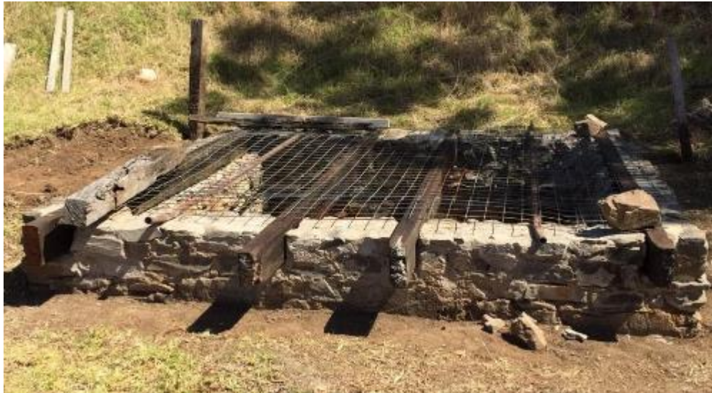
Restoration of Mary's Well
